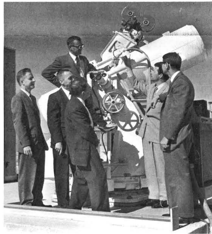
This is a cinetheodolite, a photographic missile tracking device, at a tracking station near Holloman AFB. Looking it over are, from left: Kodakers Spangler, Otto, Litten, Goldsmith (on the platform); Ward W. Topping, photographic supervisor of Land-Air Inc., and McCoy of Kodak.
