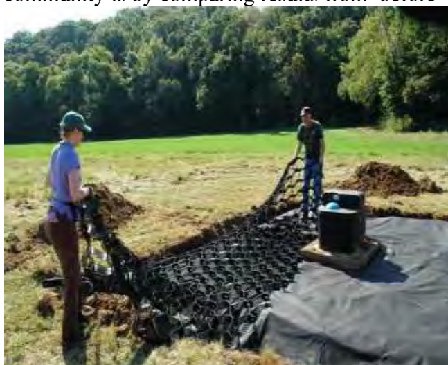
Installing a stabilized alternative livestock watering system in SCWW.
