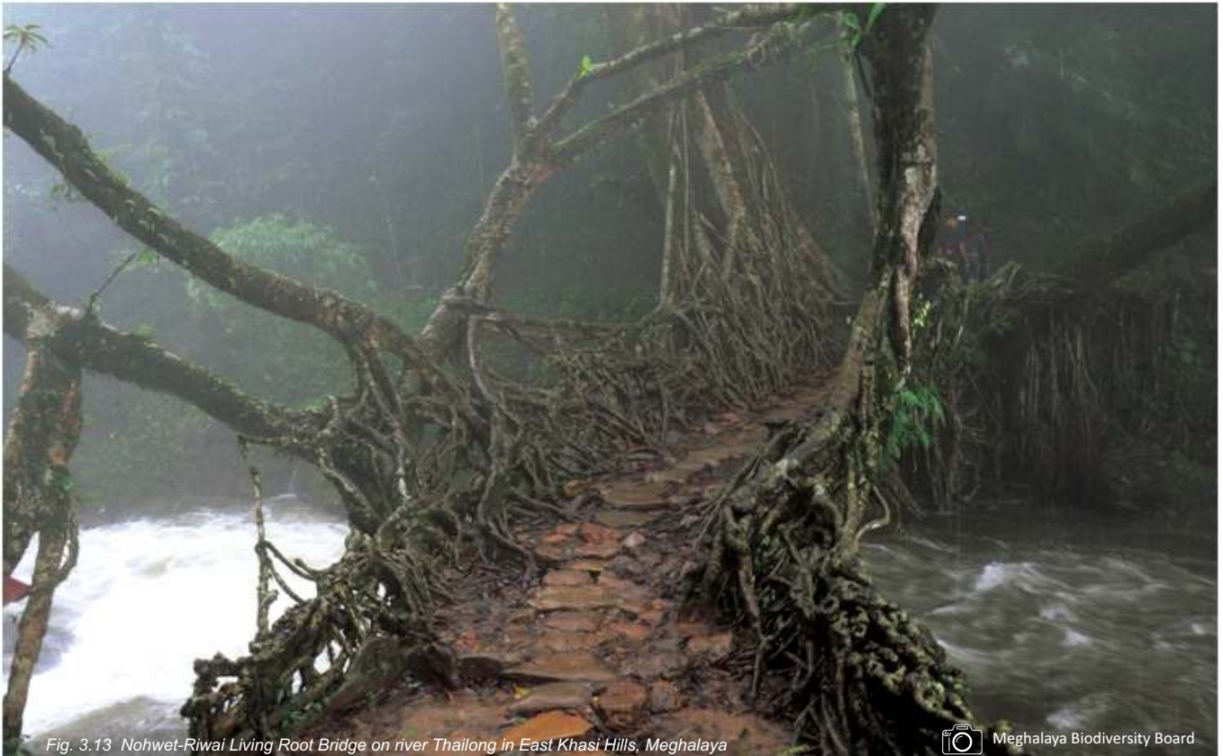
Fig. 3.13 Nohwet-Riwai Living Root Bridge on river Thailong in East Khasi Hills, Meghalaya
