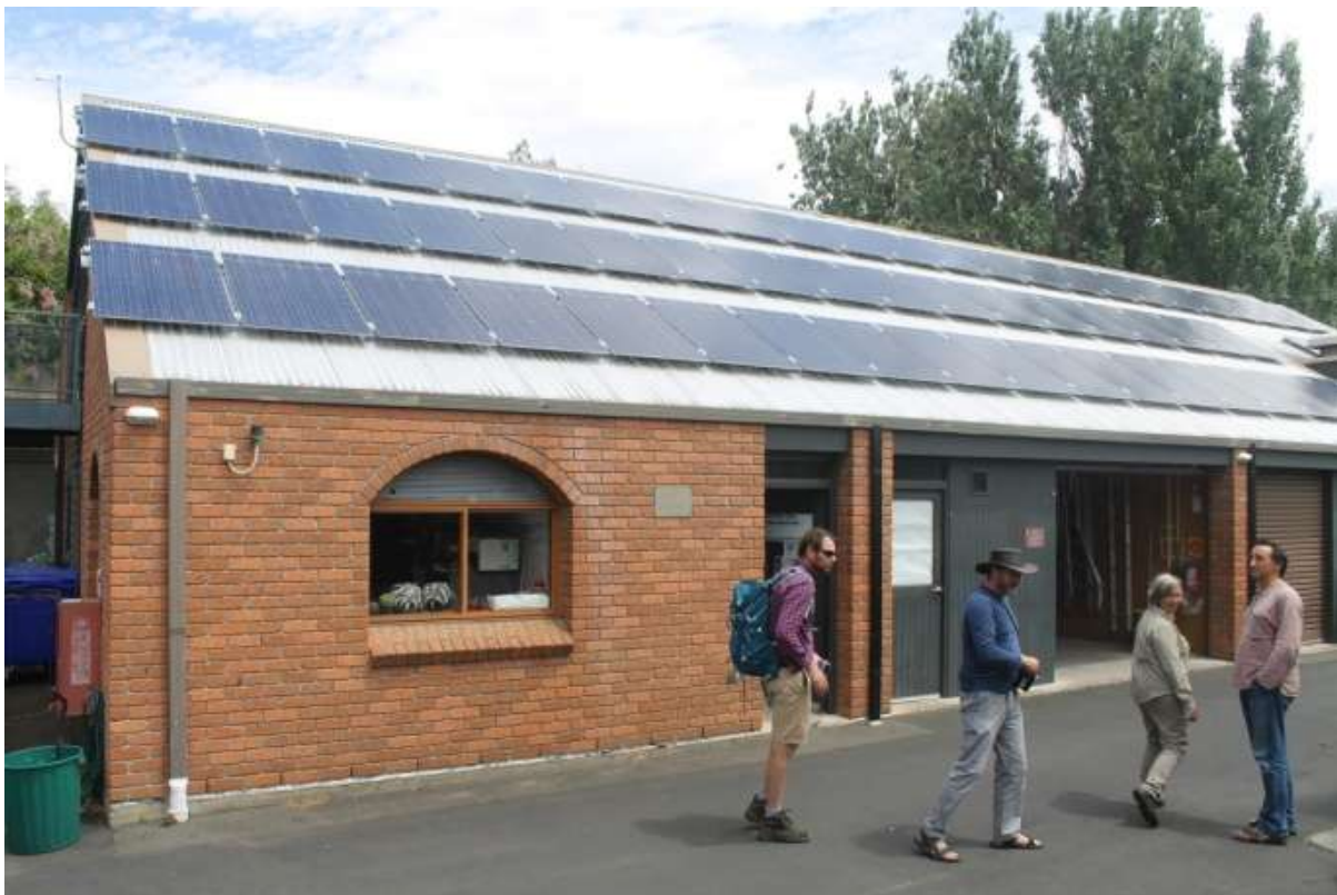
The Tasmanian Seed Conservation Centre – note the profusion of solar panels on the roof
