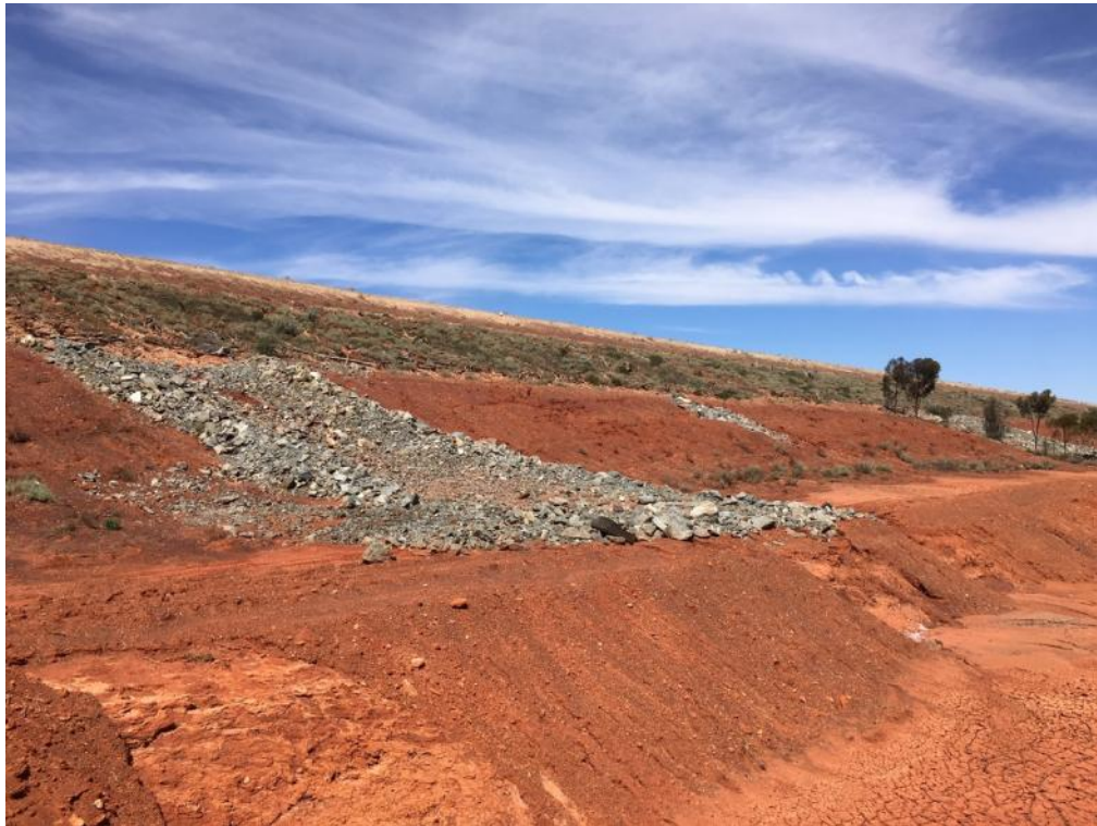
Figure 14 - Establishment of rock drains in erosion gullies on Paddington TSF 3
