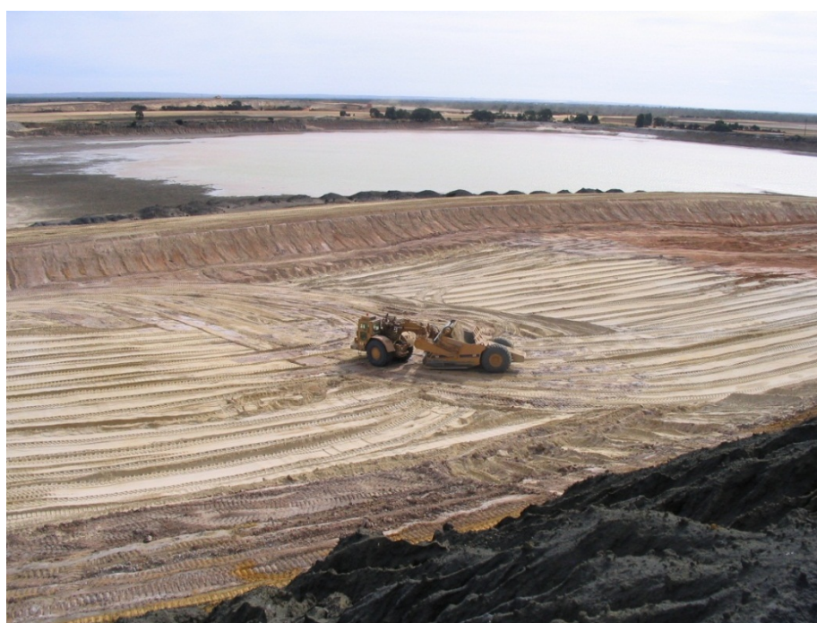
Figure 7: Construction of Waste Cell (2005)
