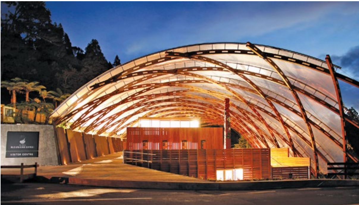
The Waitomo Glowworm Caves Visitors Centre: engineered timber was used to construct the curved roof.
