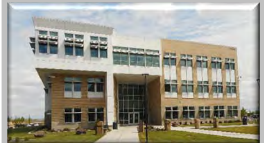
Benton County Administration Building
