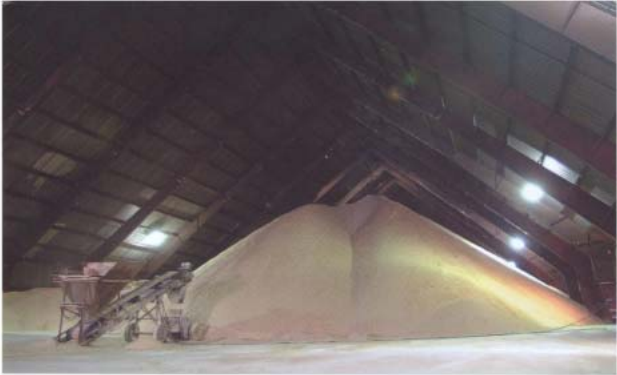
Figure 3.19. Bulk Raw Sugar Storage. This scene is within the St James Sugar Cooperative warehouse in St. James, Louisiana. Photo by John Wozniak, Louisiana State University Cooperative Extension. Used by permission.
