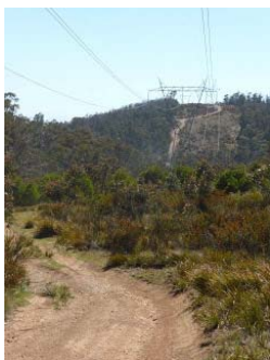
Under the powerlines Image by Martin Butterfield
