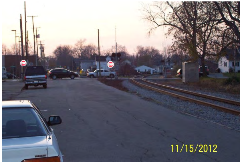
Photo 18: 2° Curve in built-up area of Van Wert, OH
