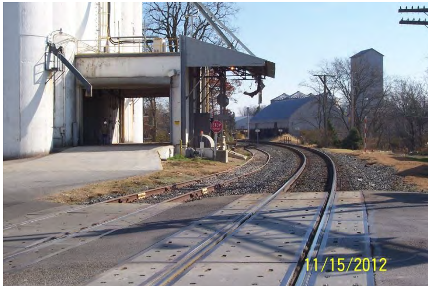
Photo 6: Single Track and Industrial Siding at North Main Street in Marysville, Ohio
