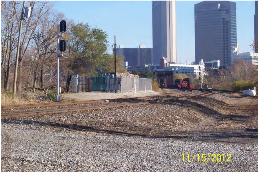
Photo 2: NS Dayton District Scioto River bridge
