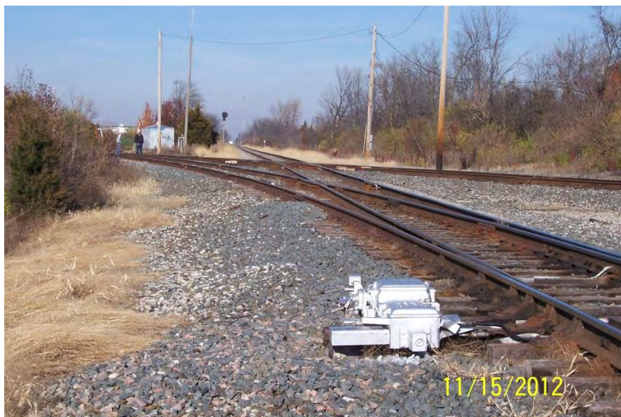
Photo 5: Diamond crossing at CP Mounds. This would be replaced by two switches to eliminate the speed restriction associated with the diamond
