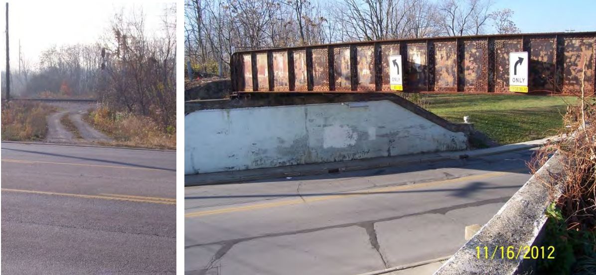
Photos 22 and 23: Abandoned NKP Right of Way crossing Jefferson Boulevard, and Abandoned GR&I Bridge crossing Main Street in Fort Wayne
