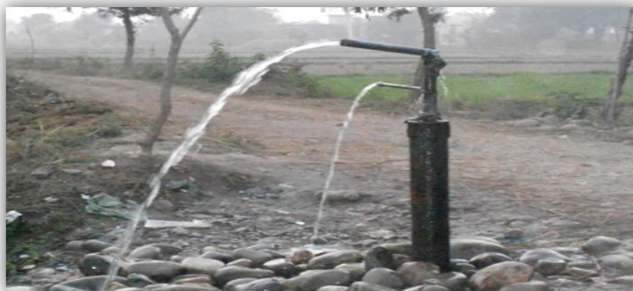
Fig. 1.1 Free flowing artesian well in Jandi area of Kathua district
