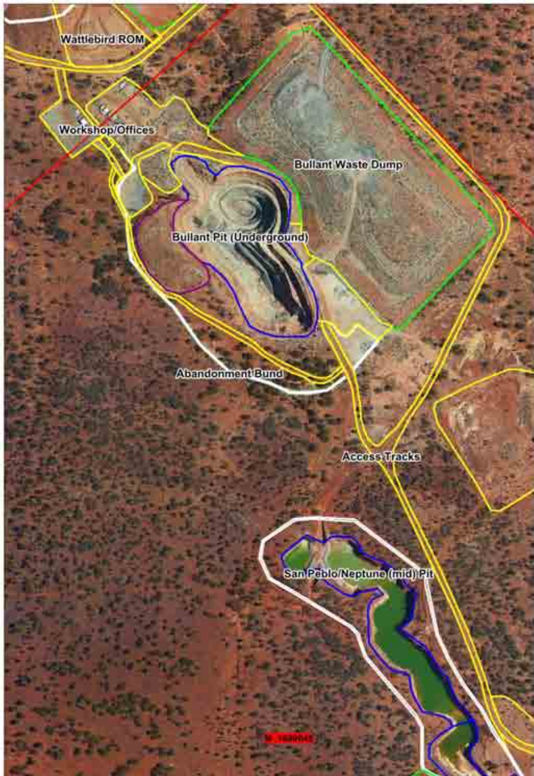
Figure 8 – Bullant Underground Operations 2016
