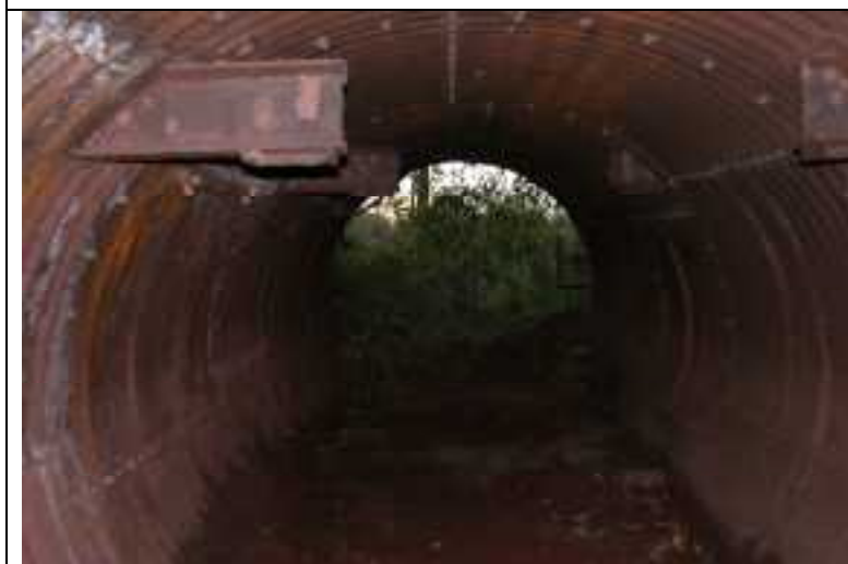
Plate 9: The conveyor tunnel where the Ghost Bats were found.
