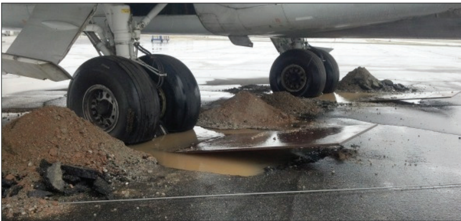
Above: A disabled B727 aircraft is parked on steel plates during its recovery process on the ramp at KRAL airport in Riverside, CA. Following the recovery, permanent concrete pads were poured for long-term parking of the aircraft at KRAL, and asphalt repairs were made to return the ramp to normal use. Image courtesy of C. Daniel Prather, Ph.D., CBU.
