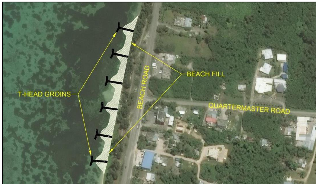
Figure 37. Beach fill project stabilized by a T-head groin field.
