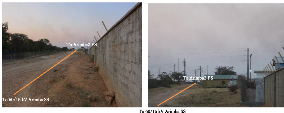
Figure 6.2-2 Local Conditions of the 60 kV Underground Distribution Line Route (Orange Line)
