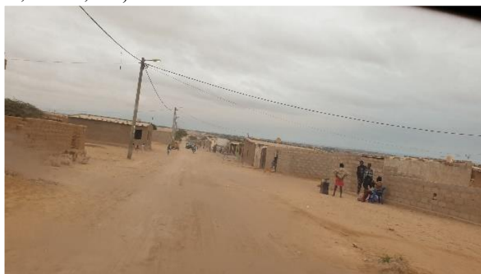
Figure 7.7-17 Condition of Road Crossing Distribution Lines to 220/60kV Namibe SS
