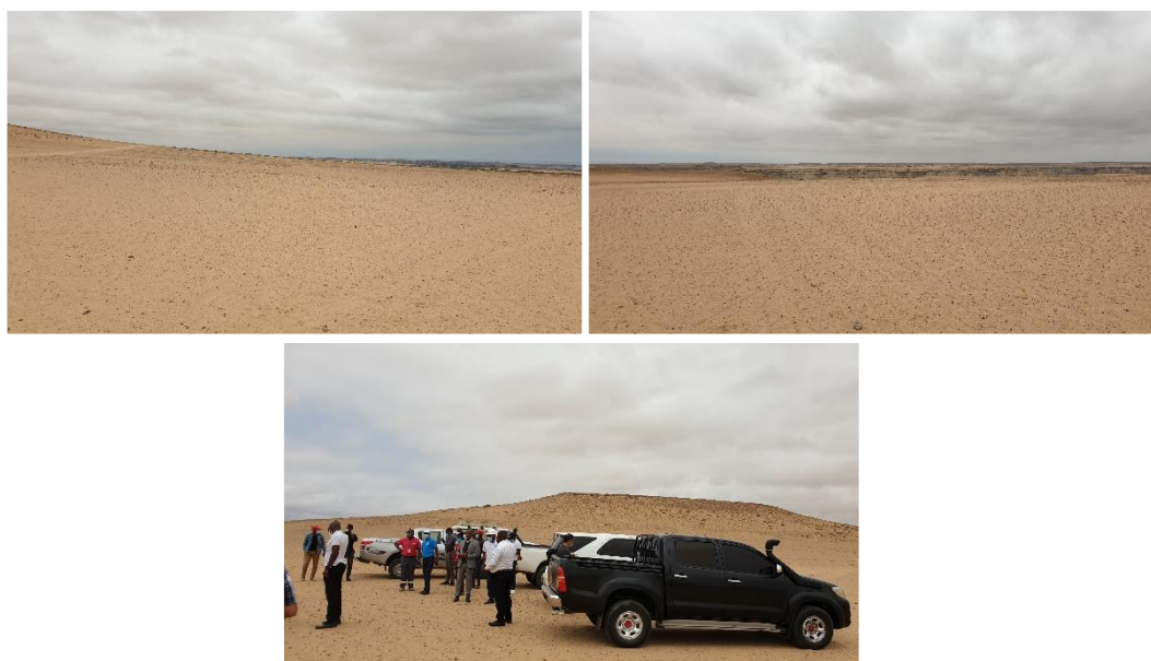
Figure 7.7-6 Situation near the proposed Namibe substation construction site
