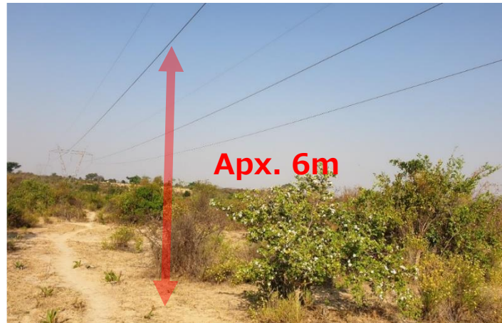
Figure 7.7-18 Status of transmission line height restrictions to the 220/60 kV East Lubango SS
