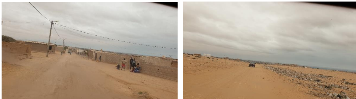
Figure 7.7-13 Condition of unpaved (left) and desert (right) roads in Namibe
