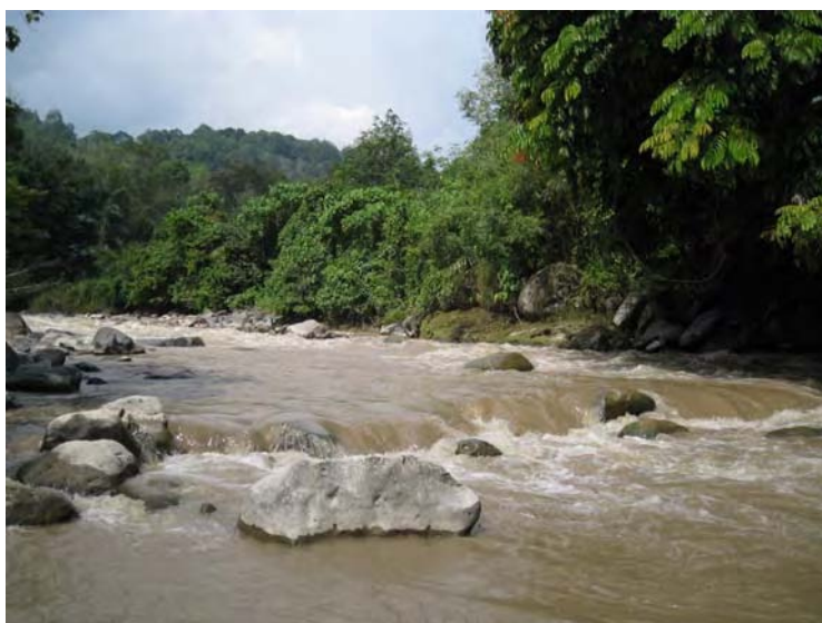
Photo 21.2.2 View of the power house point from 2km downstream
