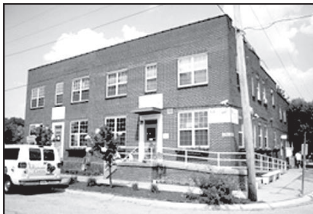
Hall Street Campus, Owensboro, Ky.
