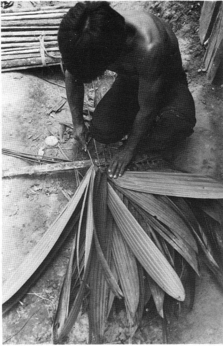
4. How leaves of "irapay" are attached on an axis made from the stem of Wettinia augusta for composing a cover unit.
