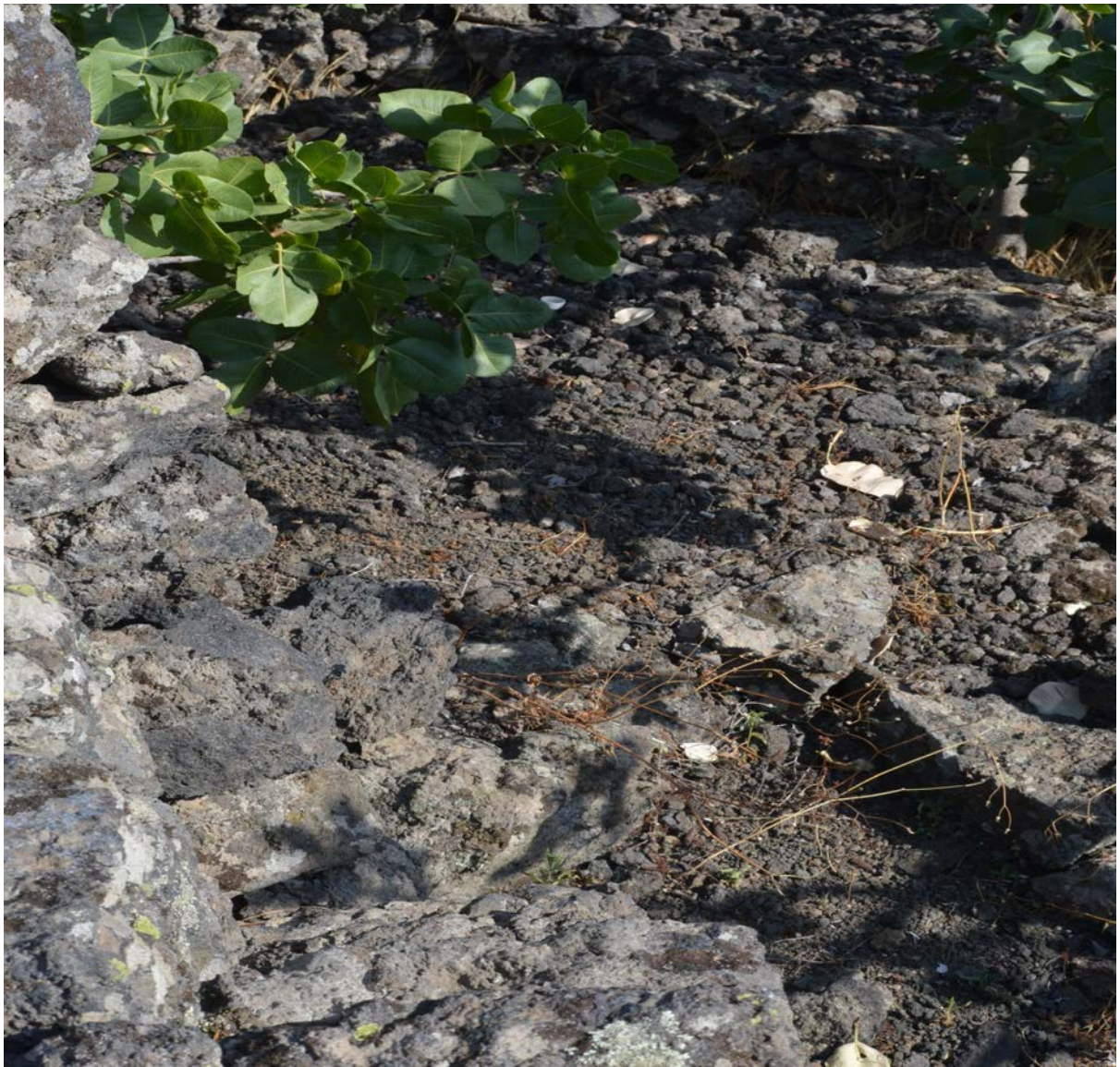
Stairs built with lava stone.
