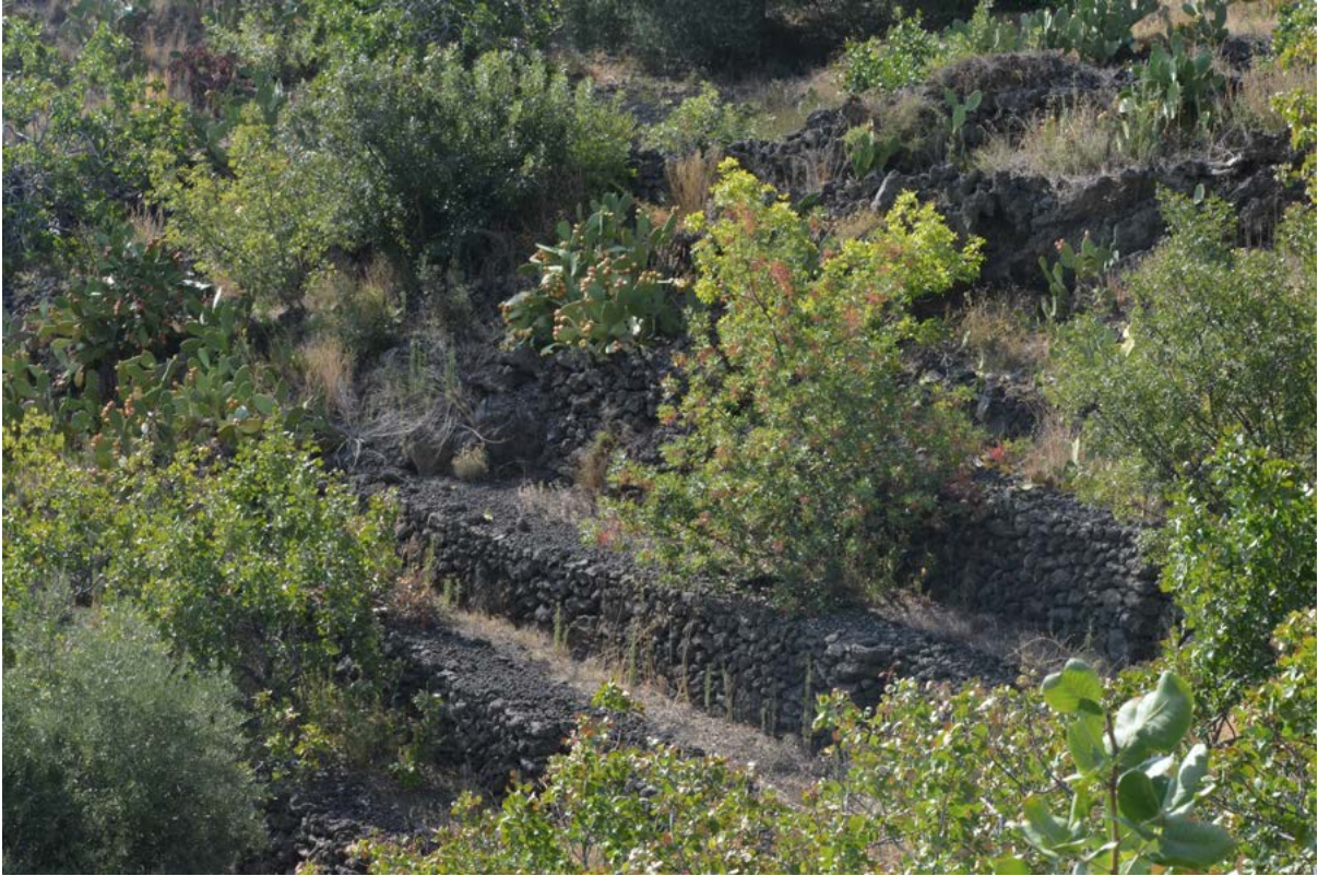
Terraces built with the dry-stone technique.
