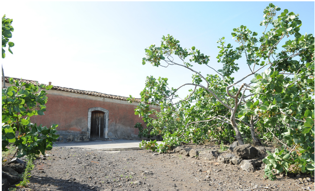
Rural building and pistachio trees.
