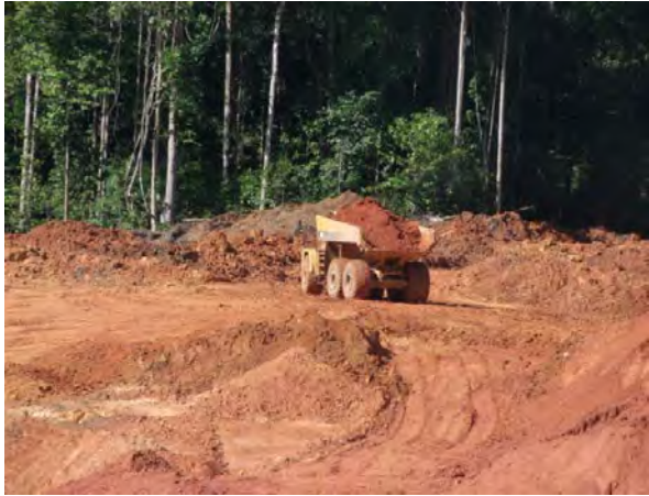
Removing laterite in Siparuni. Photo: Benn 2013
