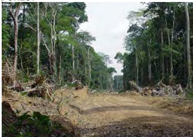
FIGURE 20: ROAD CONSTRUCTION IN CENTRAL AFRICA’S TROPICAL MOIST FOREST
