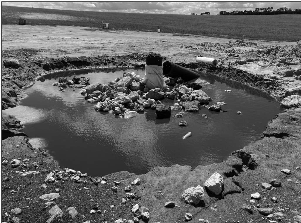
Figure 2. Sump under construction at Kimba 2.
