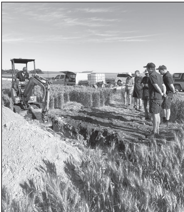
Digging a soil pit at Brimpton Lake for soil characterisation, 2021.
