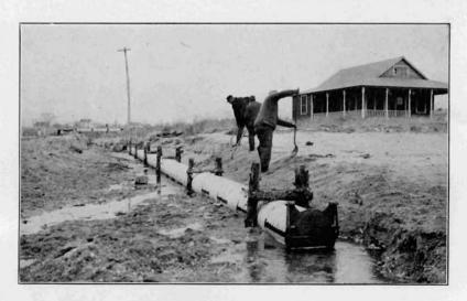
c. Installing a metal culvert through a sand beach to drain the marsh beyond, Westbrook.
