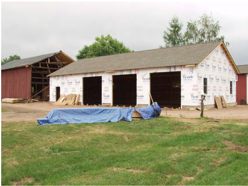
Repair and replacement of the Valley Lab damaged tobacco shed.
