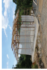
(g) Upscaling of the solar-drying cabinet to a solar-drying house. Credit: L. Jousim
