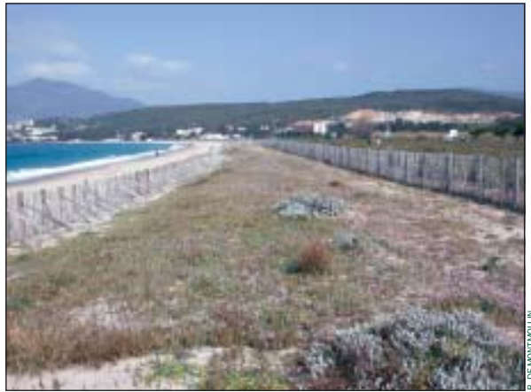
Protection of the shore above high water level, Ajaccio, Corsica.
