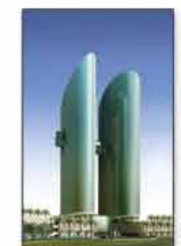
Turnkey design contract and delivery of machinery for a 1200 space Robotic Parking System for the Emirates Financial Tower in Dubai, UAE.
