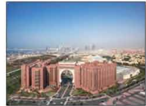
Turnkey system design, start up of operations and maintenance for a 765 space automatic parking garage for the Ibn Battuta Gate project in Dubai, UAE. Operations started in August 2009.
