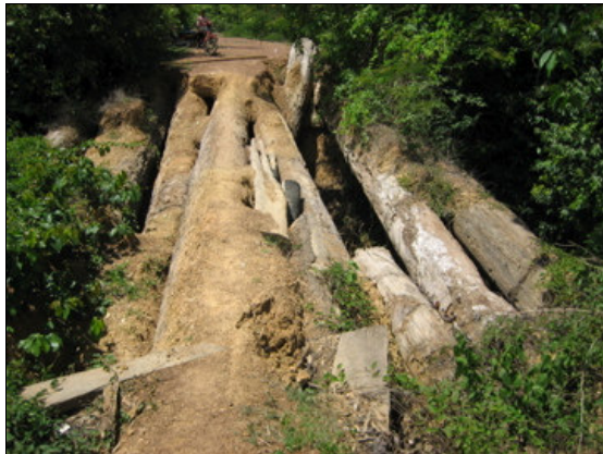
An old bridge originally used for logging
