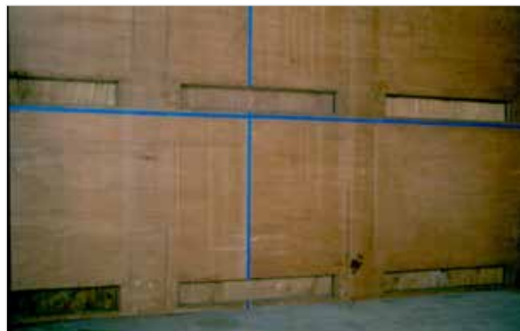
65 Front view showing 'letter boxes' (slots) in a drying wall
