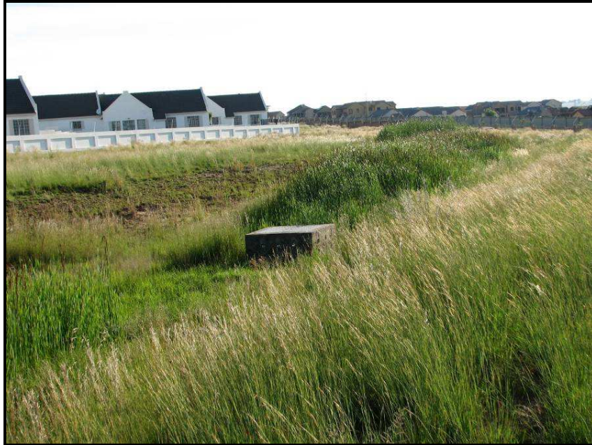
Photograph 6: Example of a swale being used in another development. This swale has been in operation for approximately 5 years and became vegetated within the first year of operation.
