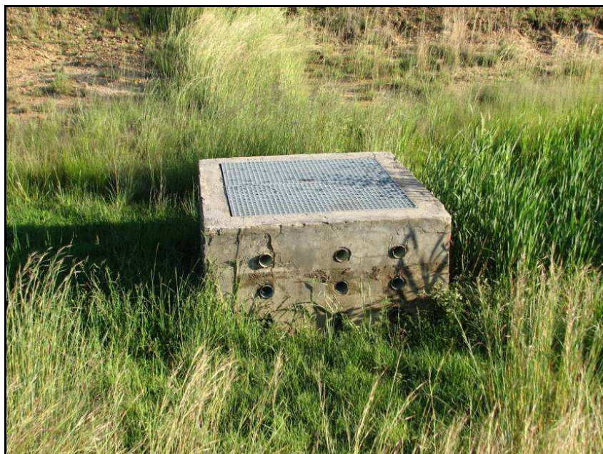
Photograph 7: Example of a drain box used in the swale above. Water drains into this box and then flows out of the swale in a controlled manner. The design of this swale also helps the deposition of sediment out of the stormwater before it enters the wetland system.
