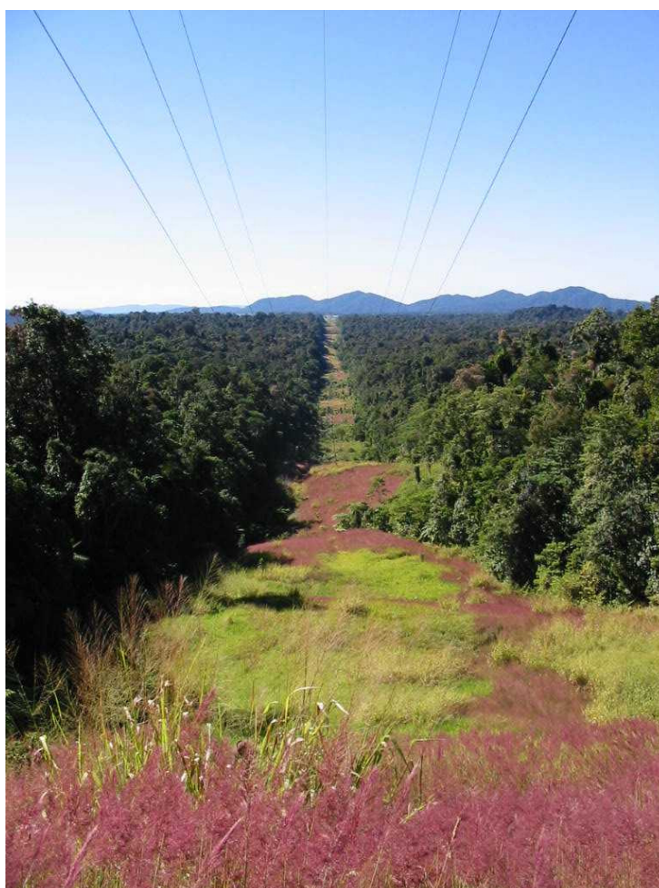
Figure 1.8: Lower section of Palmerston powerline clearing illustrating swathes of molasses grass (purple flowers), signal grass (bright green in foreground) and Guinea grass (taller pale green in foreground). Note small amounts of regrowth in gullies in middle distance.
