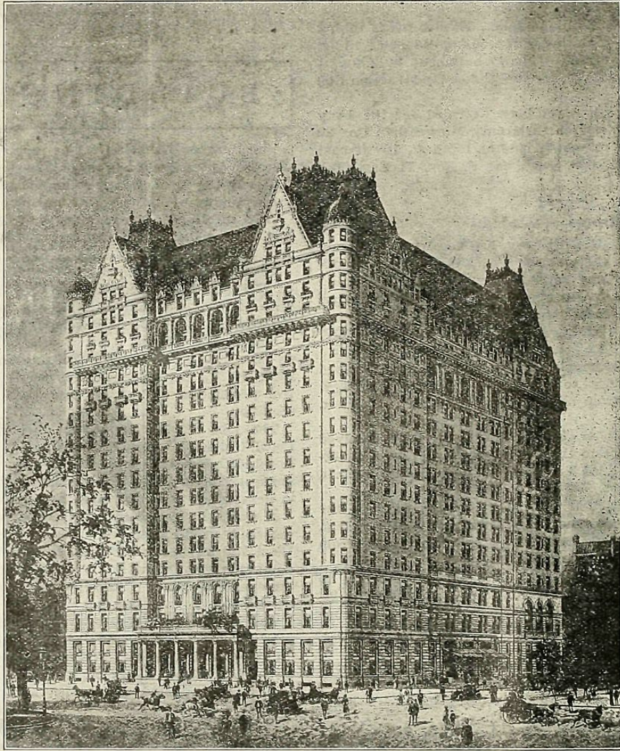
THE NEW PLAZA HOTEL. (Now in course of construction.)
