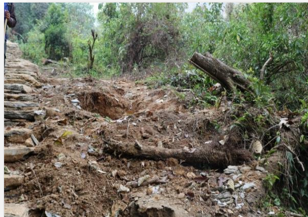
Tree fern individuals deforested due to the construction of trail affecting tree fern in Panchase Area, Nepal
