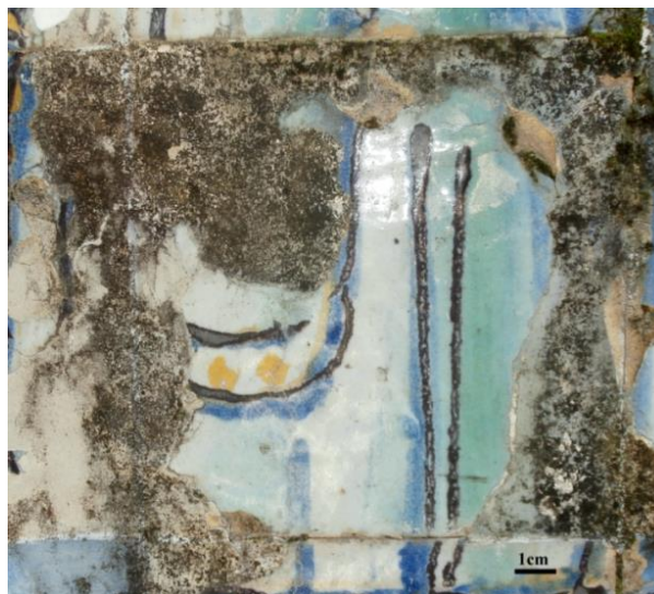
Fig. 8.3 Microbial colonization on the filling paste of glazed tiles from Marques de Fronteira Palace (Lisbon, Portugal).
