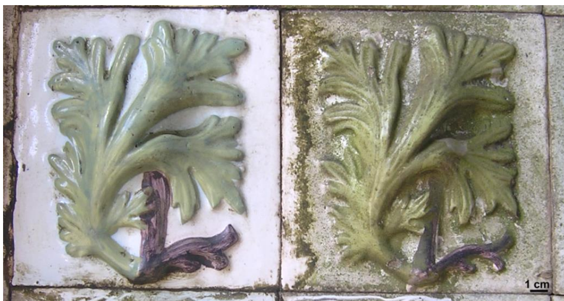
Fig. 2.7 Glazed wall tiles from Pena National Palace in Sintra (Portugal) showing a tile after the biofilm removal (on the left) and a tile covered by the green/black biofilm (on the right).
