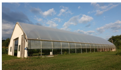
A well-cleared base-board / ground interface. Minimal space for harborage.
