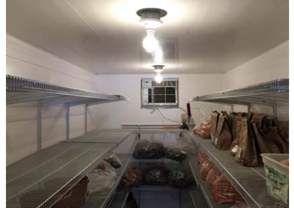
This cooler space was finished with Trusscore PVC panels resulting in a smooth, cleanable surface.
