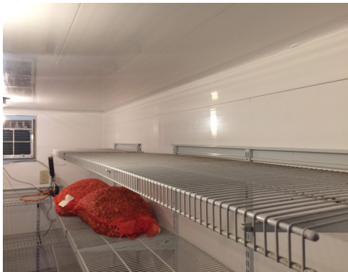
Smooth, clean and shiny, this CoolBot™ cooler used TrussCore™ twinwall PVC as a finish surface.
