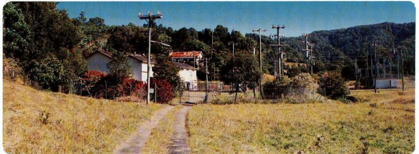
Mullumbimby Power Station
