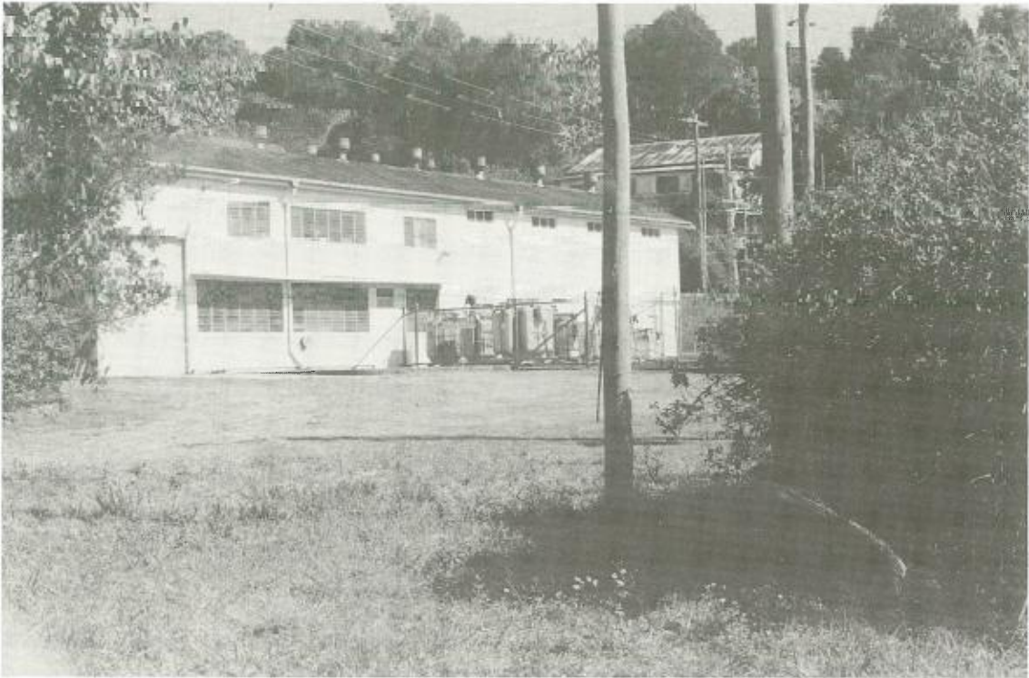
Photo 10: Mullumbimby Power Station (Area 9)
