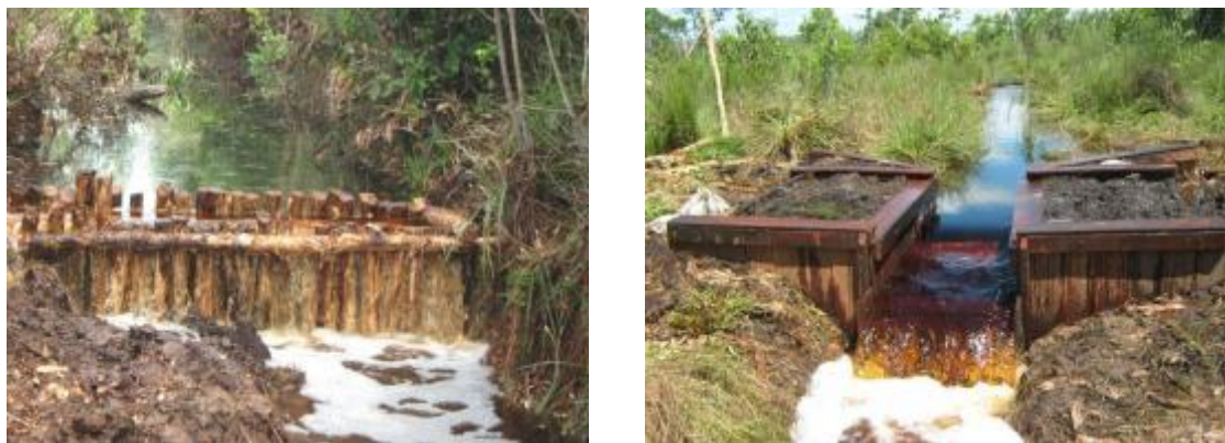
Figure 23 Simple dam (on the left) and permanent dam (on the right)
