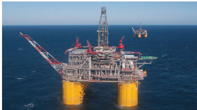
Shell's Olympus TLP on the Mars B Field in the GoM is shown with the original Mars facility in the background. The operator has applied lessons learned from building and operating its seven existing deepwater facilities in the GoM to substantially reduce development costs on its next two deepwater fields due onstream, Stones and Appomattox. (Source: Shell)
