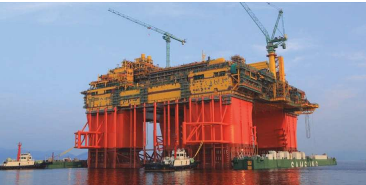
Inpex Corp. has ticked off another construction milestone at its Ichthys project after launching its CPF. (Source: Inpex)
