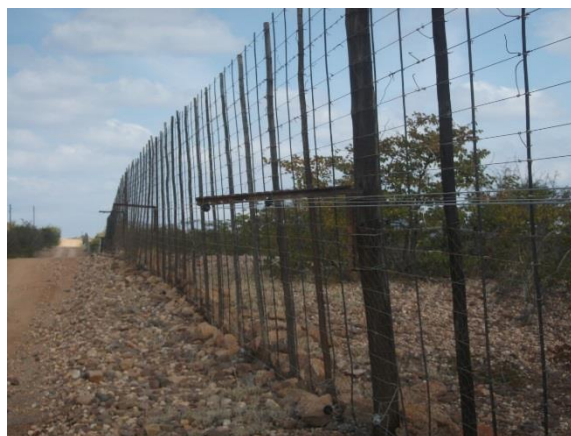
Figure 7-8: Leopard proof game fence, notice the anti-climbing shock lines.
