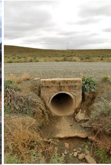
Plate 2: existing pipe culvert
