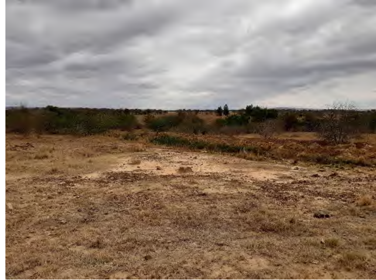
Stormwater drainage channel from pivots south west of the dam
