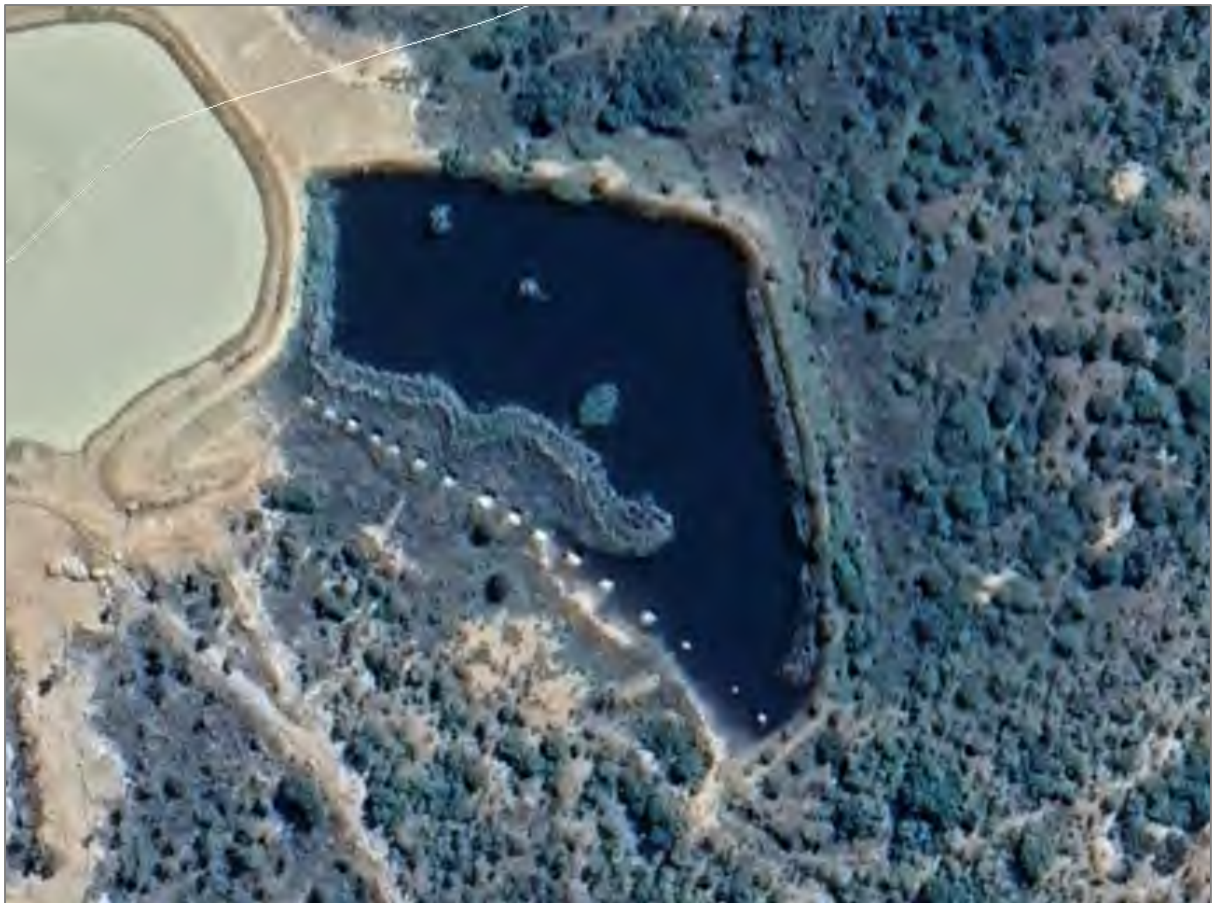
Figure 11-6 Off stream water storage facility(Google Earth Imagery,2019)
