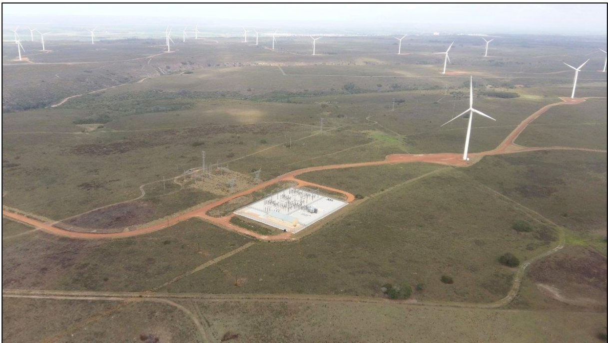
Figure 3. On-site substation of the Jeffreys Bay Wind Farm which would be similar to the on-site substations required for the Impofu Wind Farms.
