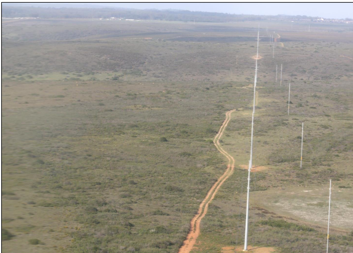
Figure 4. Example of 132 kV power line which would be similar to the current project, showing the extent of the pylon footprint areas, access road and the likely impact associated with the construction of the current power line.
