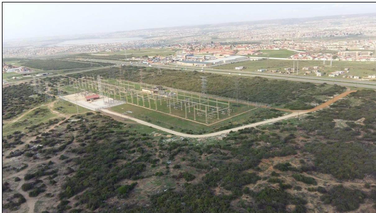
Figure 36. Aerial view of the Chatty substation, with the R75 and Kwadwesi township in the background. There is some remnant thicket around the substation, but overall, this area is considered low sensitivity due to the large amount of transformation and urbanisation this area has experienced. Common species in this thicket include Portulacaria afra , Euclea undulata , Cussonia spicata , Aloe speciosa , Schotia afra var. afra , Carissa bispinosa subsp. bispinosa , Grewia occidentalis , Putterlickia pyracantha , Sarcostemma viminale , Optunia ficus-indica , Asparagus multiflorus and Sansevieria aethiopica .
