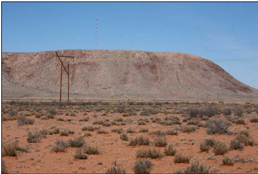
Figure 5. Looking from next to the existing Eskom substation towards the Gamsberg, where the power line will cross the N14.
