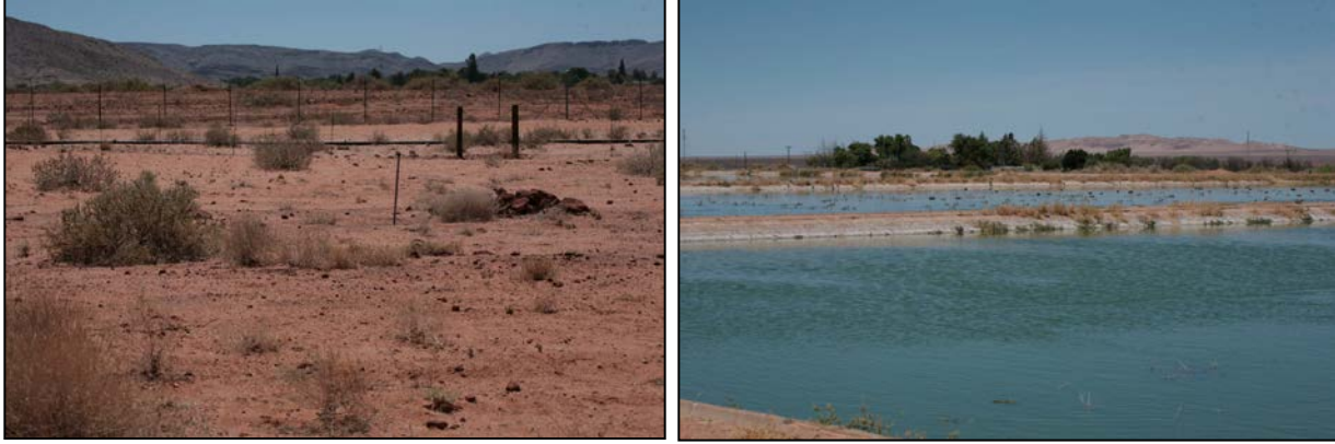
Figure 3. The expansion area for waste water treatment works and a section of the existing works.
