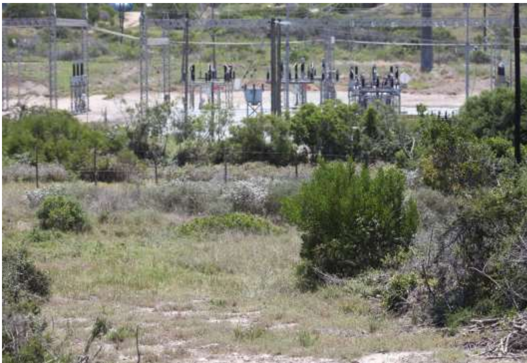
Photo 4 Part of site in foreground and substation adjacent to the northern part of the site opposite the road in the background. Photo: R.F. Terblanche
