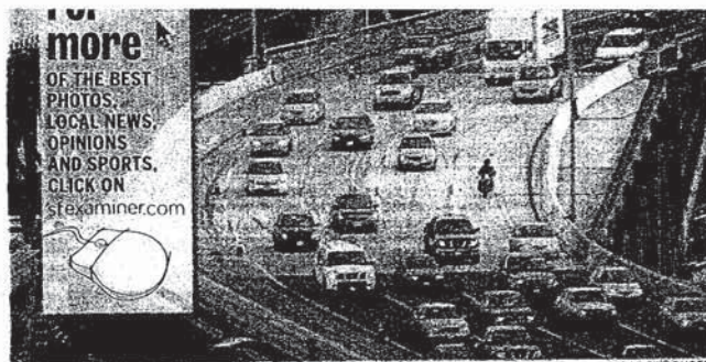
Deadly curve: The Bay Bridge S-curve was the site of a fatal accident Nov. 9, when a truck traveling 50 mph flipped and plummeted off the road, killing the driver.
