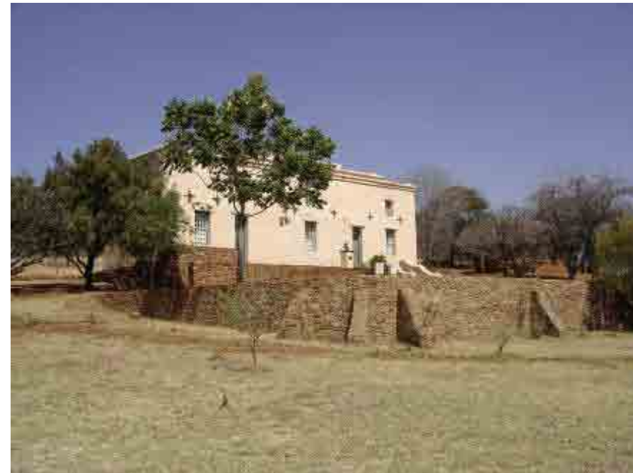
Figure 8-5: Main house on Boekenhoutfontein, President Paul Kruger's farm in 1873-1900, a provincial heritage site managed by a private hotel group
