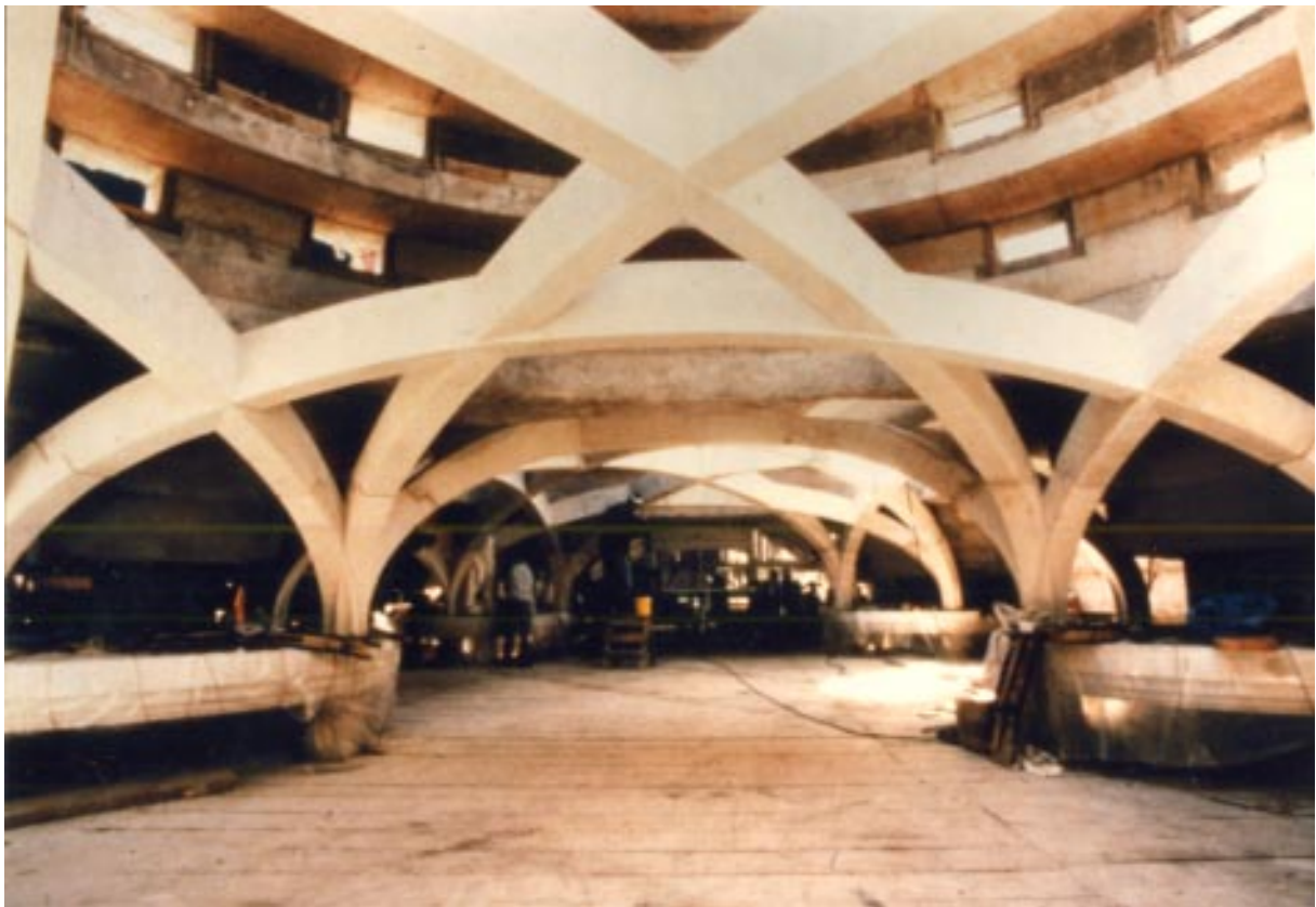
The Mosque during construction
